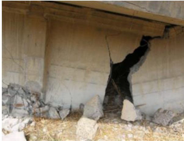
ID-4.2 Bridge beam: mid span fracture (Anania et al, 2018).
