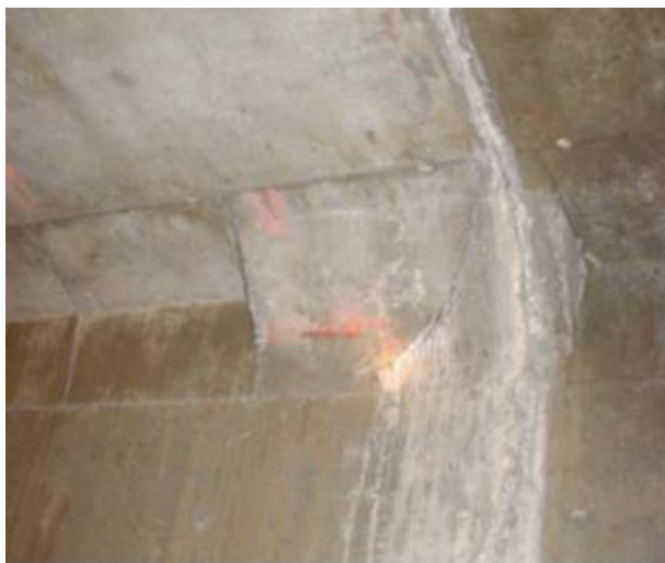
ID-14.3. View of a crack showing effervescence (Reis, 2007).
