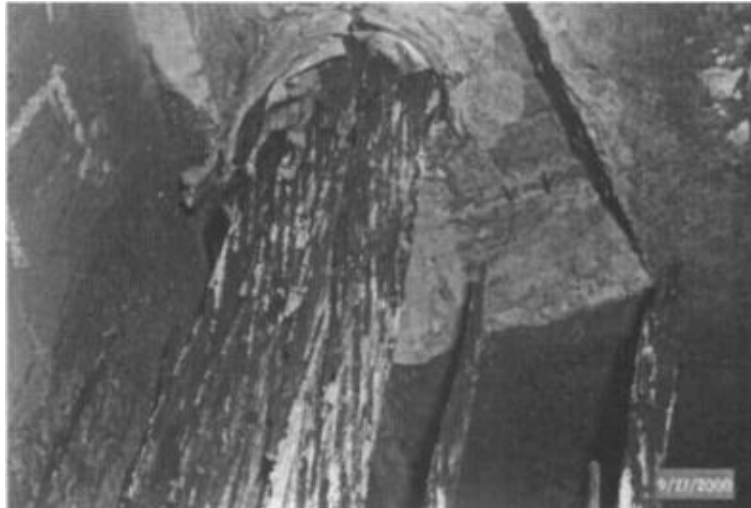
ID-11.5. Severe corrosion and failure just below the cap on the SE tendon in column 133 NB (Theryo et al, 2011).
