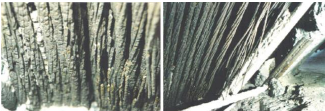
ID-6.6. Details of top part of the suspension cables, strongly corroded in 1991 (Nuti et al, 2020).
