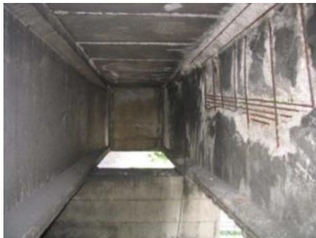
ID-21.6. Damage observed on internal surfaces of the prefabricated beams in 2006 (Di Prisco et al, 2018).
