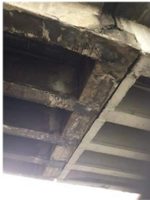
ID-21.8. Critical dapped-end joint view before the collapse: bottom view (Di Prisco et al, 2018).
