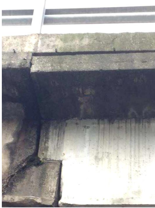
ID-21.7. Critical dapped-end joint view before the collapse: side view (Di Prisco et al, 2018).
