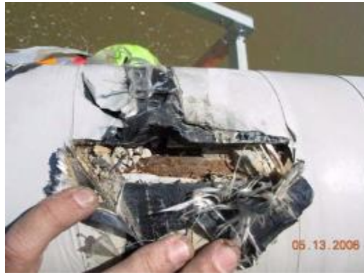
Figure 3.3.6. Luling Bridge (ID-10). Corrosion of wires at PE split (Mehrabi, 2009).
