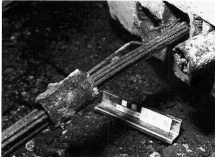
ID-1.4. Metal sleeve over longitudinal tendon: corrosion of tendons at joints (Woodward and Williams, 1988).
