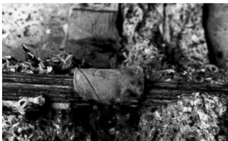
Figure 2.2.6. Cardboard tube across transverse joint in Ynys-y-Gwas bridge (ID-1) (Woodward and Williams, 1988).
