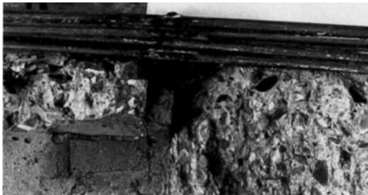
ID-1.5. Longitudinal tendon crossing a transverse joint: corrosion at localized joint (Woodward and Williams, 1988).
