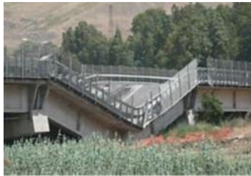
Figure 3.1.8. Collapse mechanism of Petrulla Viaduct (ID-4) (Anania et al, 2018).
