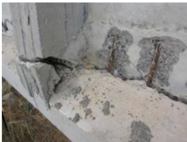
ID-4.9. Detailed view of vertical mild reinforcement expelled by the rotation of the lower flange (Anania et al, 2018).
