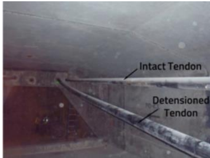
ID-15.4. Detentioned PT Tendon discovered in July 2011 (Ahern et al, 2018).
