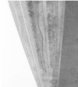
Figure 3.1.17. Lowe's Motor Speedway (ID-9): longitudinal crack in double-T stem directly under the grout plug location (Poston and West, 2005).
