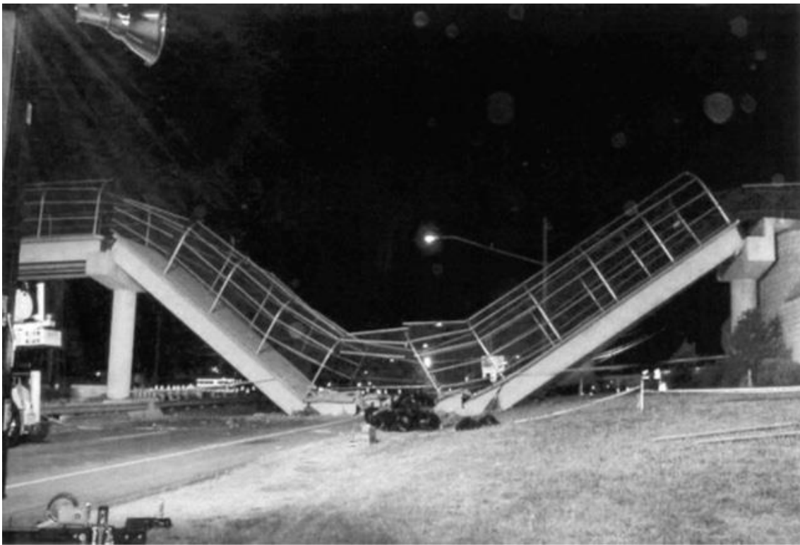
ID-9.1. Collapsed span of pedestrian bridge (Poston and West, 2005).
