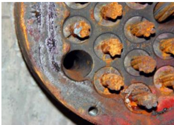
ID-14.1. Close-up view of an anchorage head at tendon location E3E-CO4S (continuity tendon) showing signs of corrosion from water collecting at the anchorage (Reis, 2007).
