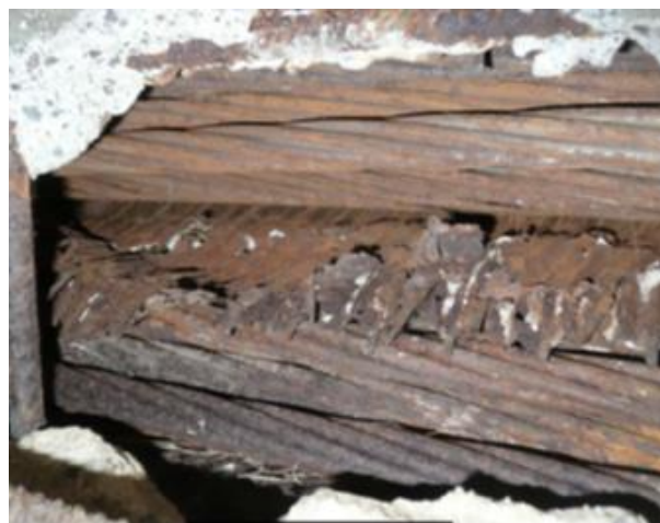
ID-4.6. Congestion of strands in the mid span of the bridge beams (Anania et al, 2018).
