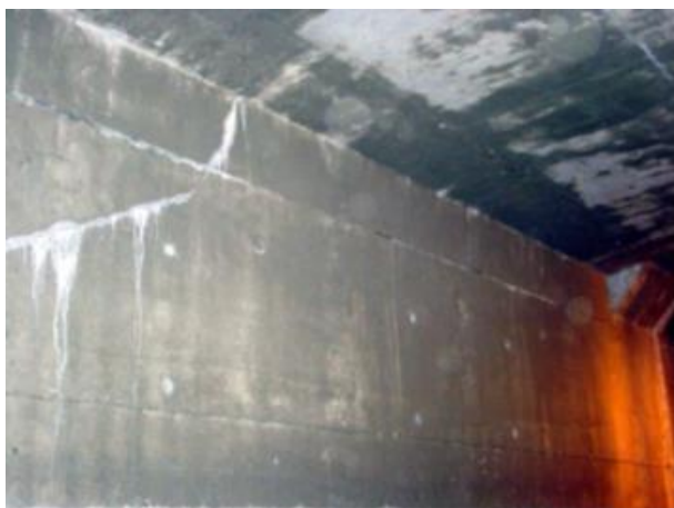
ID-14.2. View of interior web wall showing a crack and effervescence (Reis, 2007).
