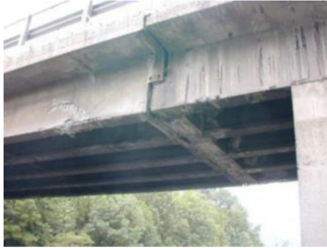
ID-21.4. Lateral impacts occurred in 2006 due to trucks circulating on SS.36 towards Lecco: location (Di Prisco et al, 2018).
