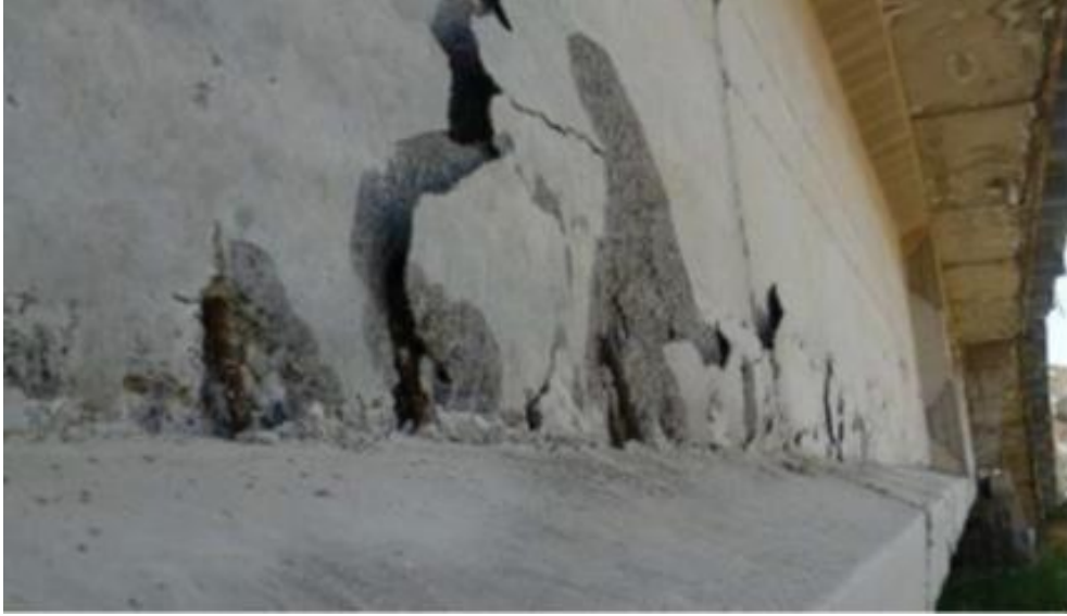
ID-4.10. Cracking on the bridge span due to tensile stress and to the expulsion of the stirrups (Anania et al, 2018).
