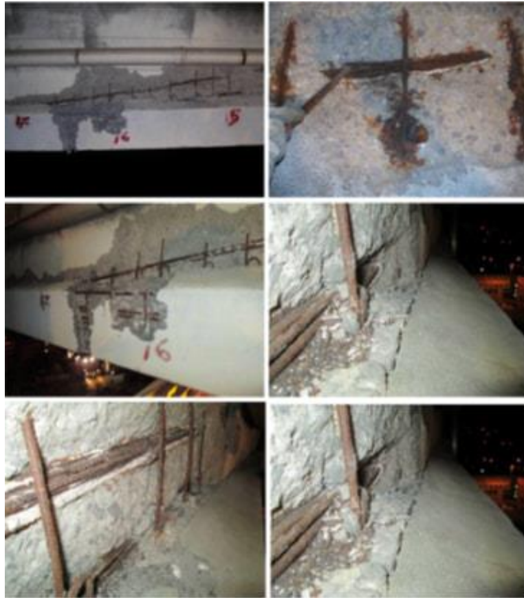
Figure 3.1.18. Polcevera Bridge (ID-6). View of cables toward the support in 2011 (top) and 2013 (middle). Zoom of the cables in 2013 (bottom) where corrosion and partial pitting can be observed (Nuti et al, 2020).
