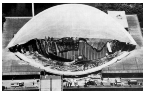
Figure 3.1.6. Berlin Congress Hall (ID-19). View from the South on the collapsed roof overhang in 1980 (Helmerich and Zunkel, 2014).
